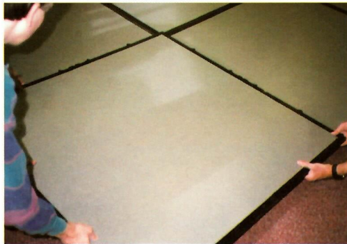
3. Pushing the Interlocking Floor Panels together
