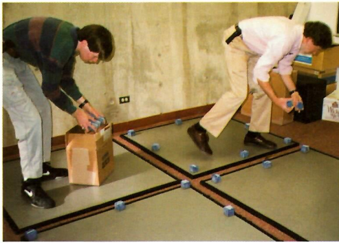
2. Laying out the Floor Panels and placing Isolation Blocks
